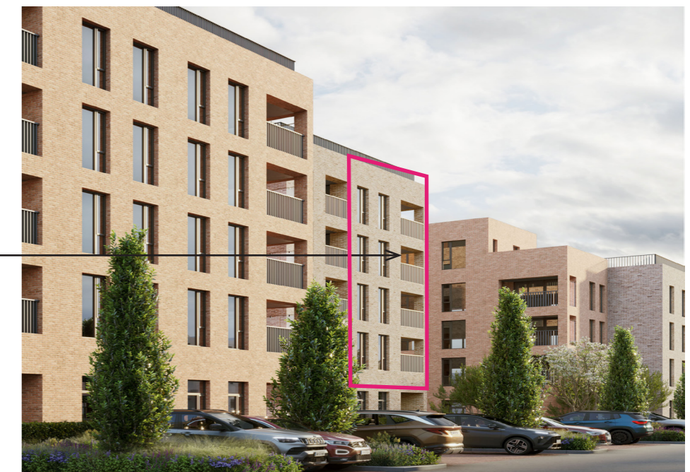
Figure A.38 - 3D Verified view along Belltree Avenue. Showing Blocks 6 facade of Units 06-01-28 ,06-02-28, 06-03-28, 06-04-28
