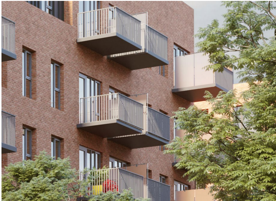
Figure 12.8 - 3D verified view of Block 5 balconies, showing the privacy screens between adjacent balconies.
