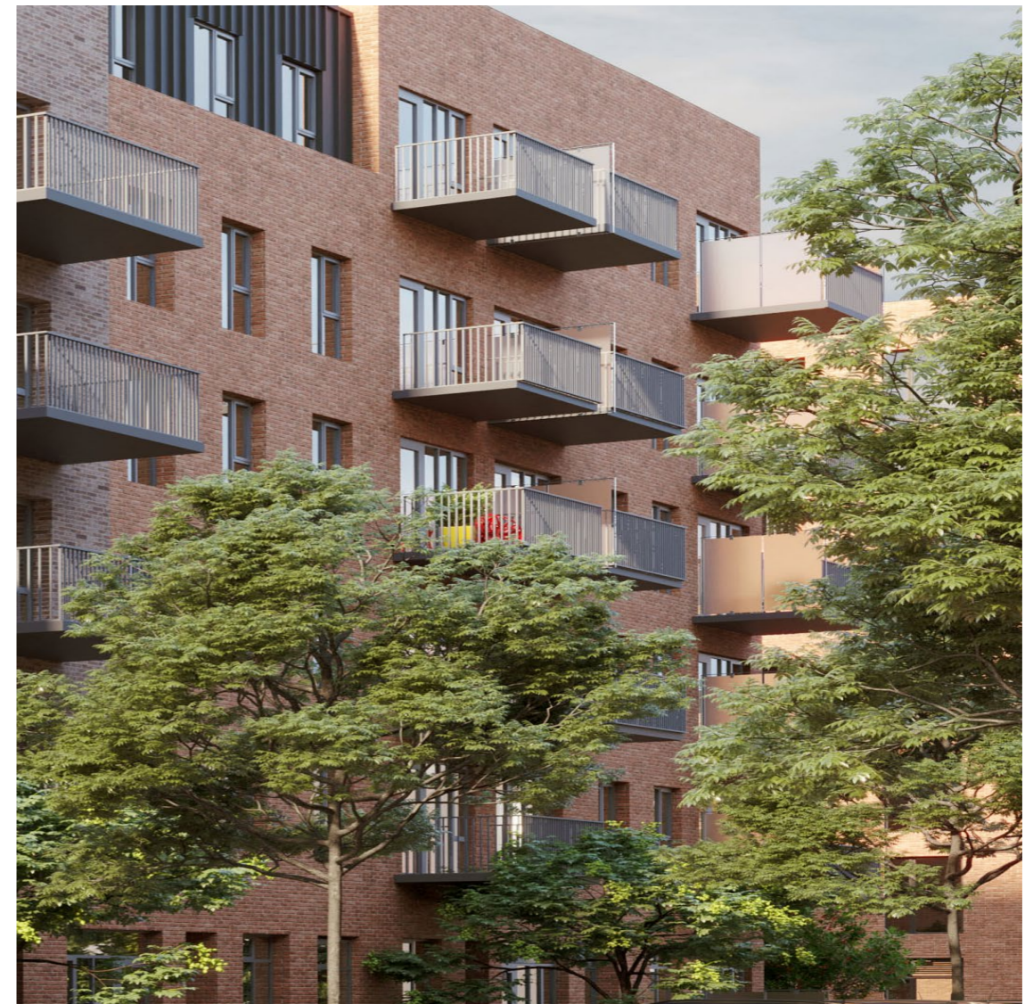
Figure 11.2 - Showing 1.8 high obscure glass privacy screens between apartments and their balconies on Block 5.
