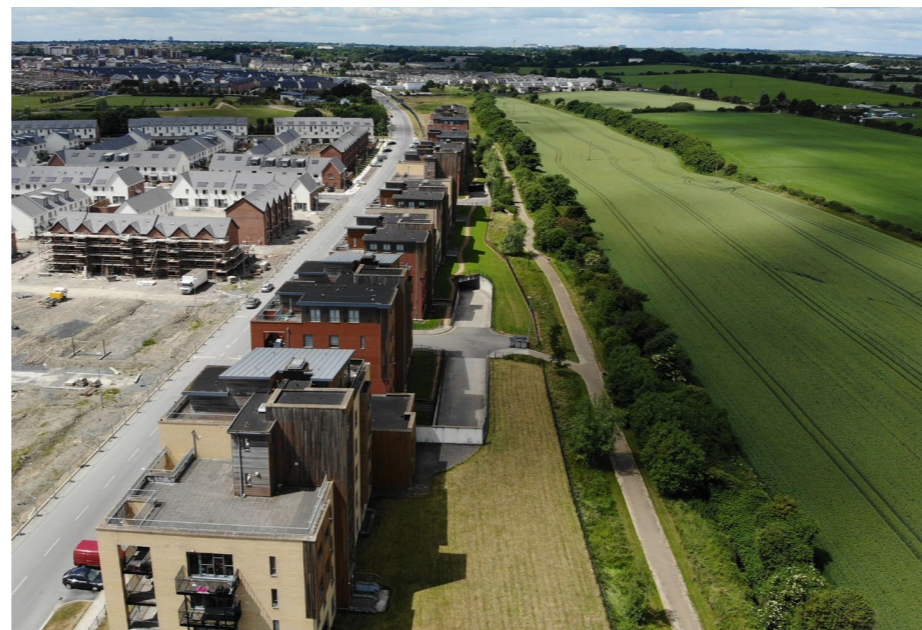
Figure 2.1 - Birdseye view of Mayne River Linear Park at the northern edge of Clongriffin
