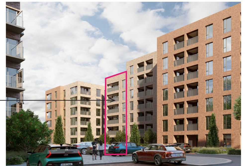
Figure A.68 - 3D verified view of Block 6 along Lake Street with facade of Units 06-00-07, 06-01-08, 06-02-08, 06-03-08, 06-04-08
