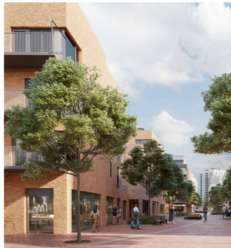
Figure 8.9 - Block 5 - view along Market Street looking east towards Station Square
