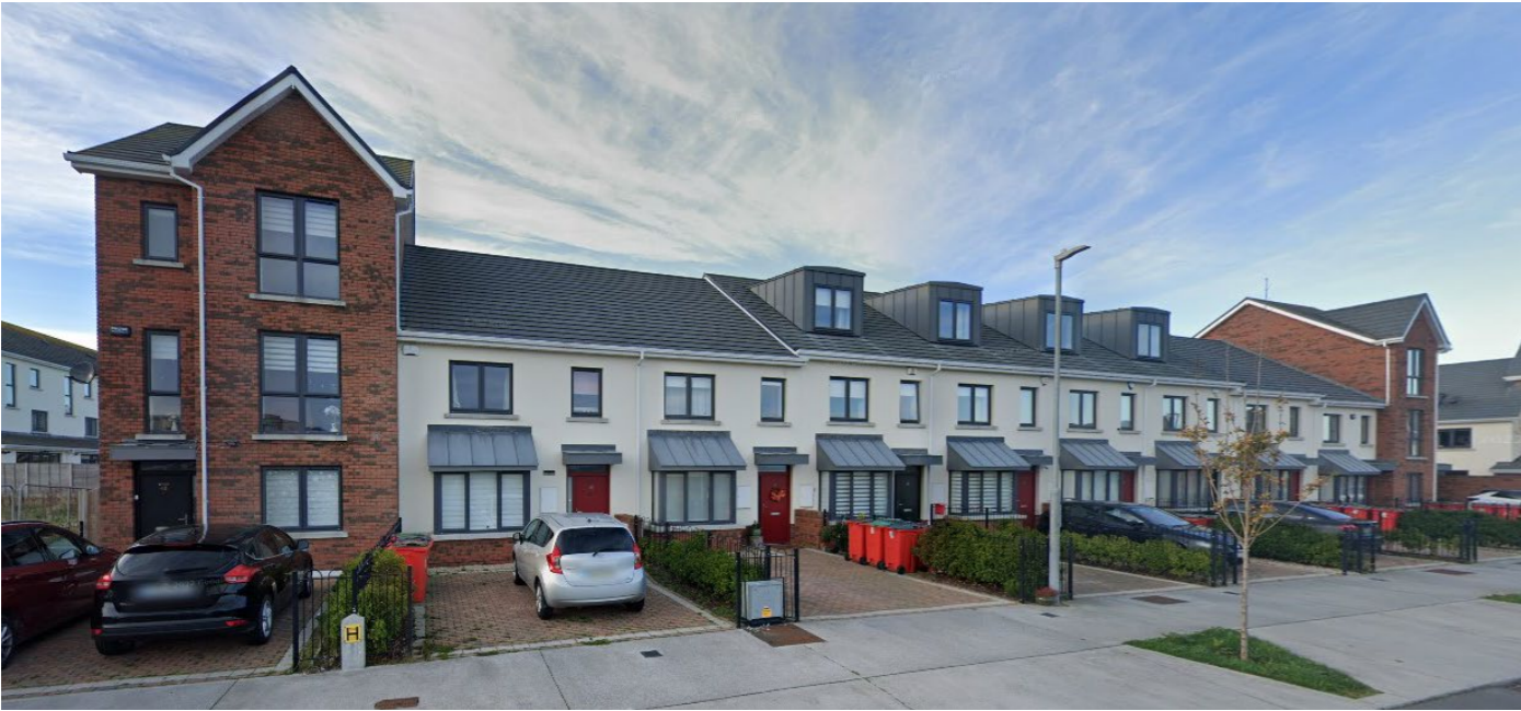
Figure 1.2 Terraced houses to the west of Block 6 on Park Street
