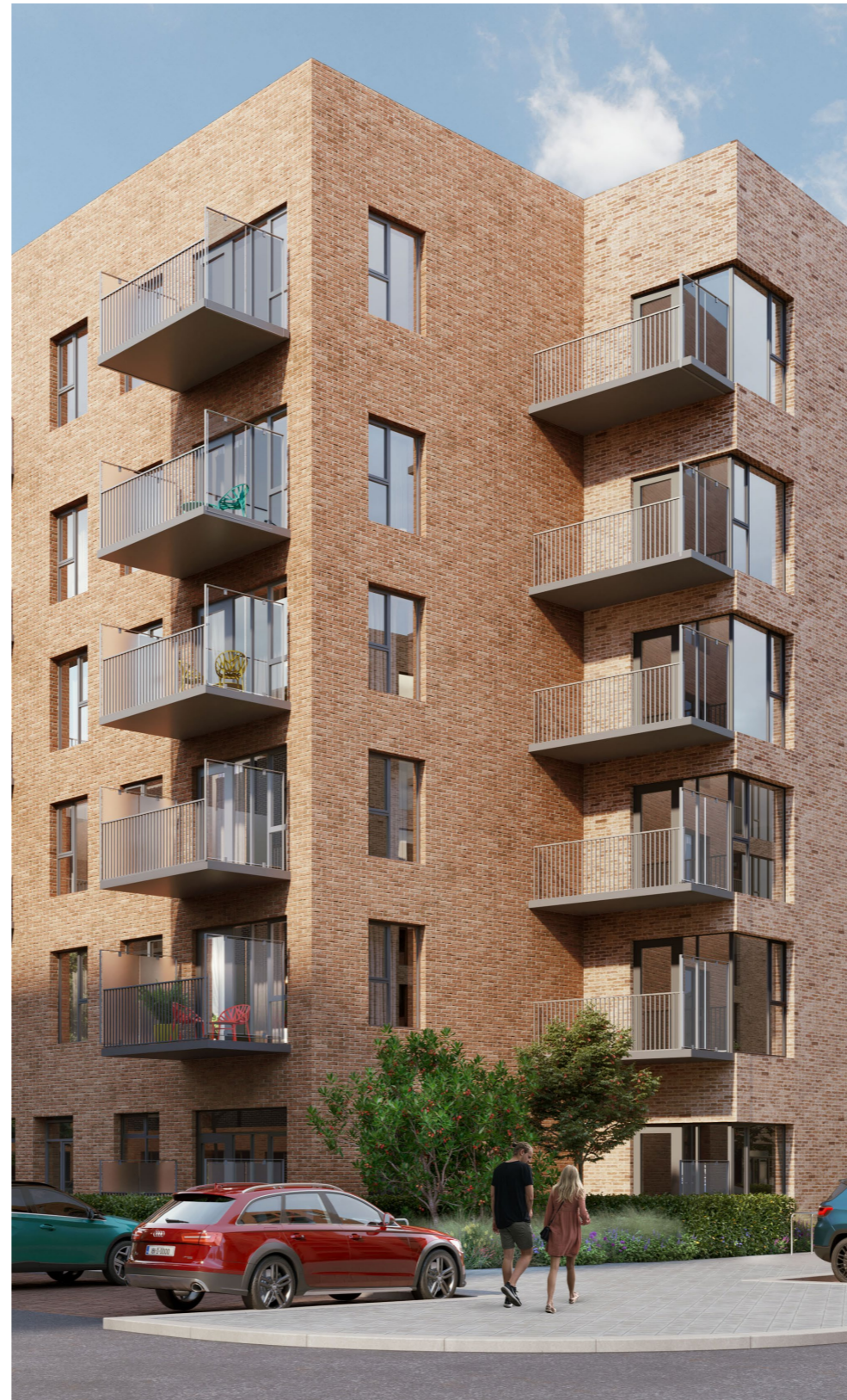
Figure 12.16.0 - Wind screens, planting and soft landscape features on the sides of Block 5's corner-facing balconies.
