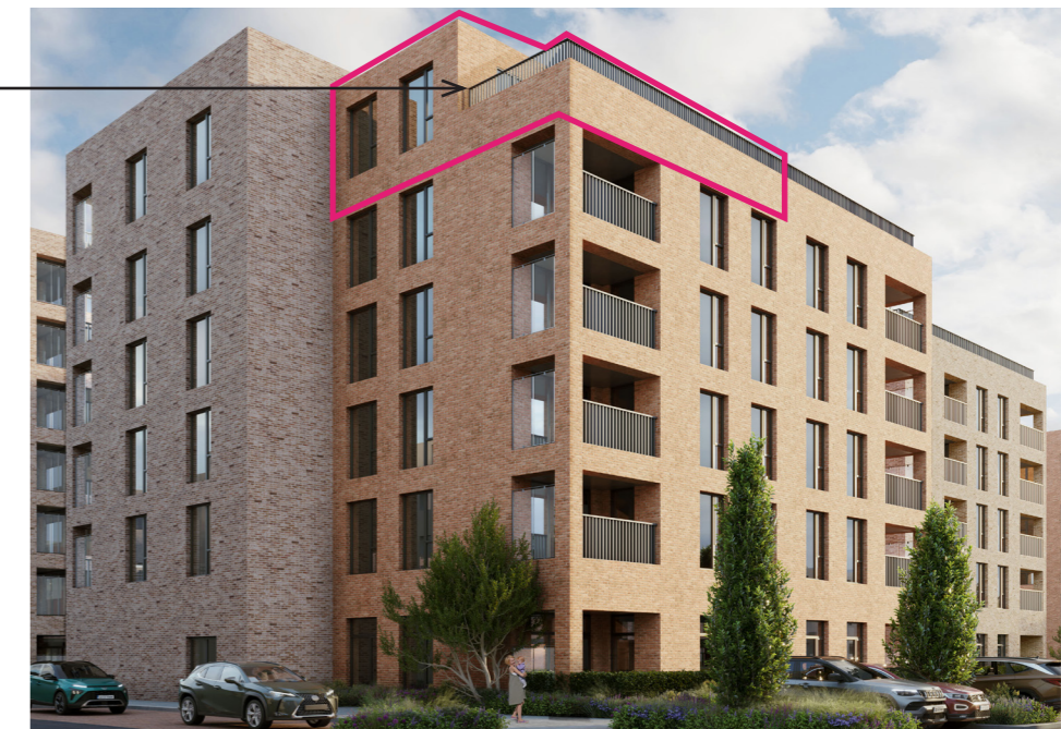
Figure A.80 - 3D verified view of Block 6 along Belltree Avenue facade of Unit 06-05-07,
