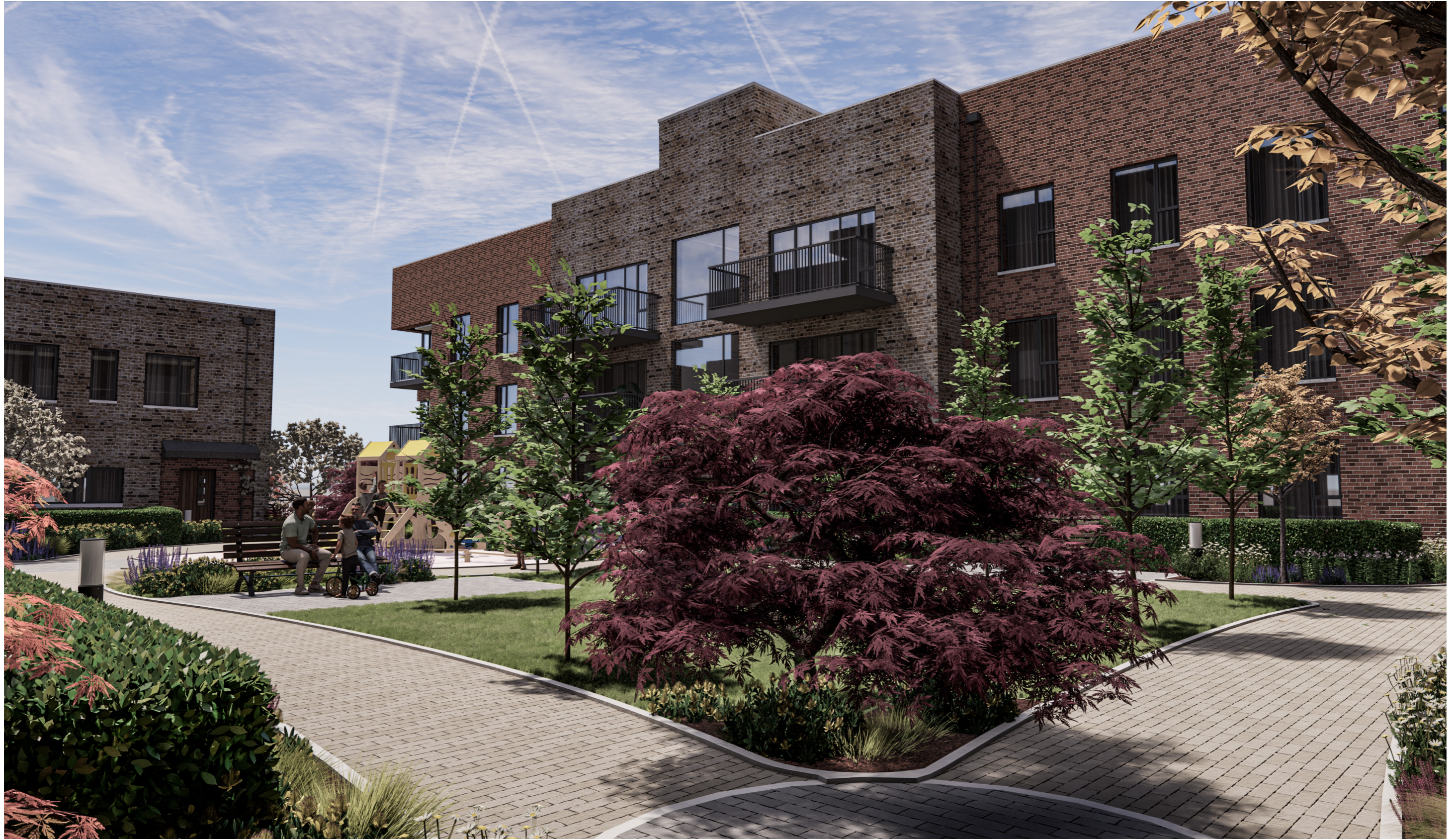
Figure A.8 - Block 5, North East of Podium looking South West
