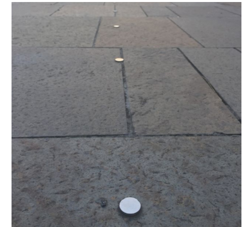
Figure 5.20 - Stainless steel demarcation studs to the perimeter of the area
