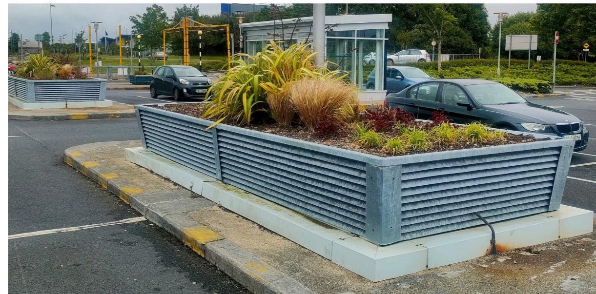
Figure 5.5 - Option 2 - Linear vent with higher upstand of 1.2m, planting on top and louvred vents to the sides.
